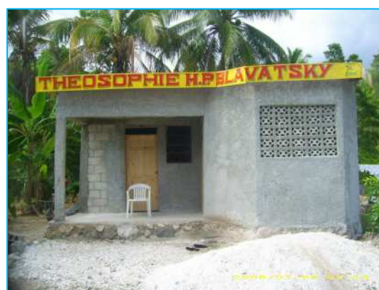
The new Lodge under construction in Jacmel, Haiti
